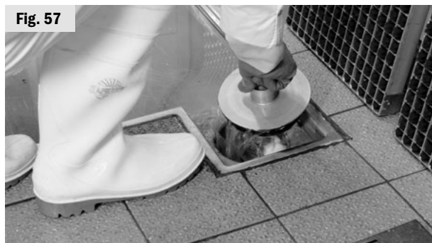
2. Remove the overflow plug to allow liquid to drain.
